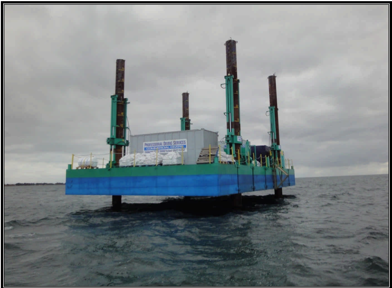
Fig. 1. Jacked up barge in position to the wreck of the Clarence. The dark blue container contains the data analysis room and the X-ray enclosure.
